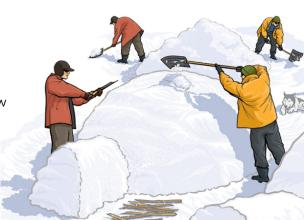
Step 2: Shape the mound into a dome and allow it to sinter for about 90 minutes. Then begin to hollow out the mound.
